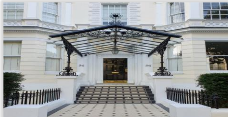
INTERNAL COMMUNAL REFURBISHMENT
